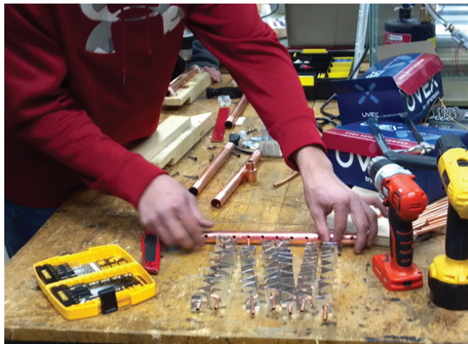
BUILD: Working on heat exchanger
